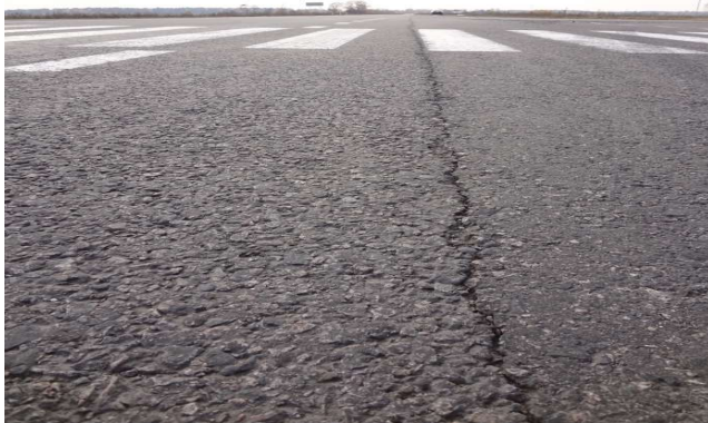
Figure 5 – Longitudinal crack along the pavement axis on the section PK 308+577 (it is seen a difference between SMA structure) modified with synthetic wax (left) and natural bitumen (right)
