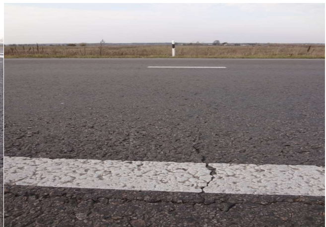
Figure 6 – Transverse crack in the SMA layer modified with synthetic wax, which is positioned perpendicular to the longitudinal crack along the pavement axis
