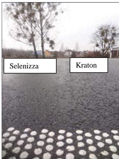
Figure 8 – Joint with SMA including Kraton (profile)
