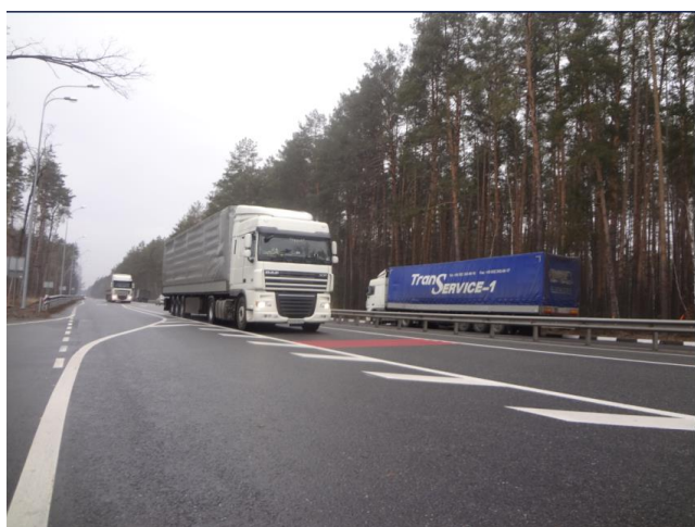
Figure 6 – General view of the ramp on PK 33+850
