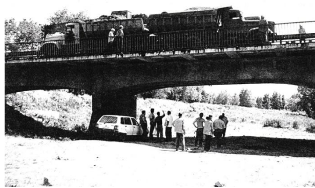
Figure 1 - Testing a bridge across the Vorskla river near the Bilyky village the Kobeliaky area after reconstruction
