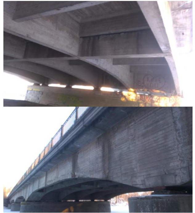
Figure 2 - A bridge across the Vorskla river near the South Station in Poltava city
