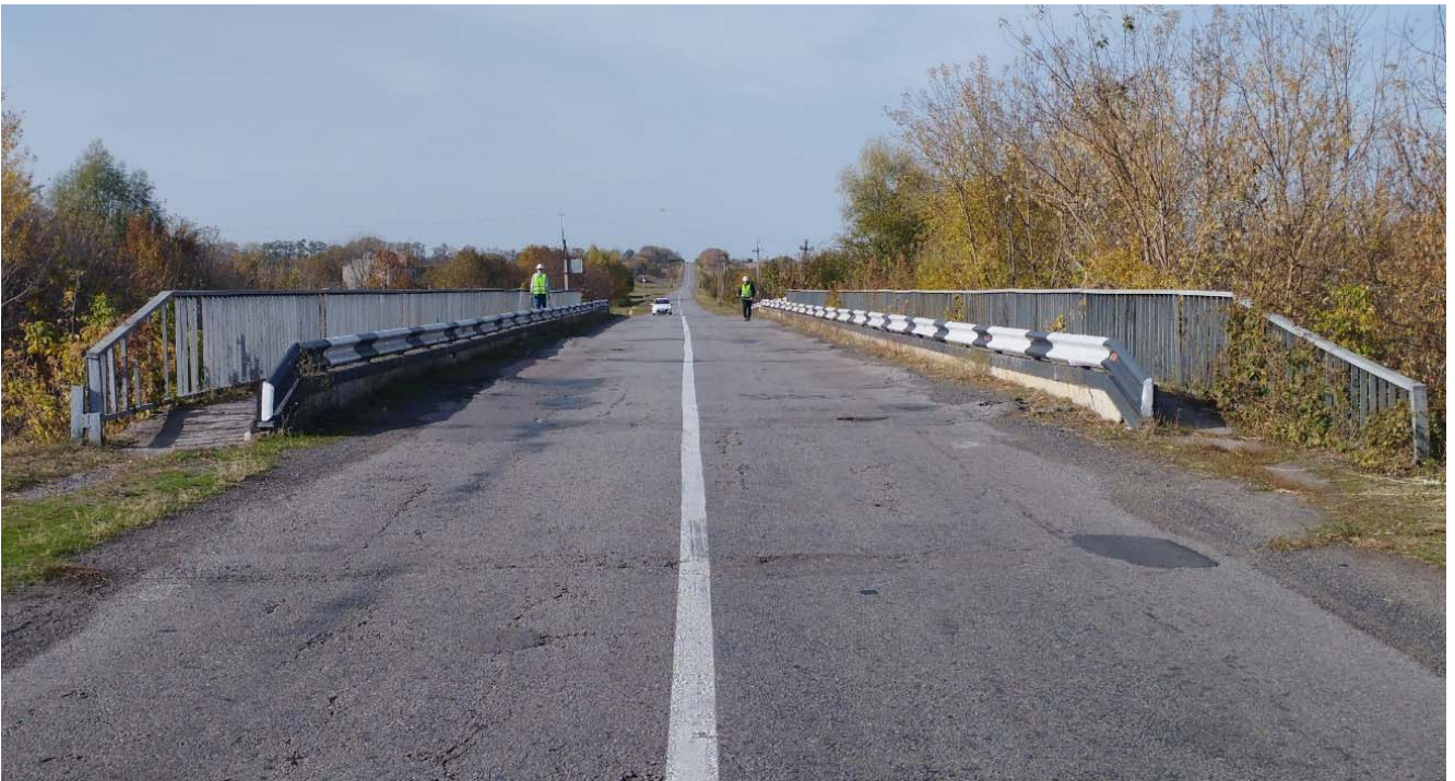
Figure 1 – Bridge crossing over the river on the A-B road section
